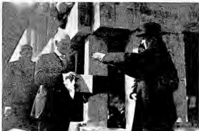
Construction of Payne County Court House
